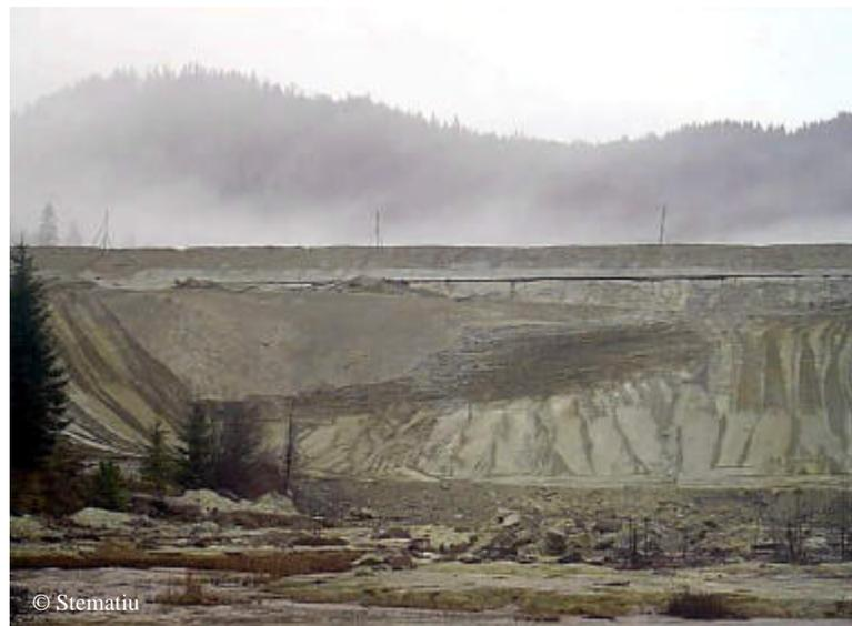
Photo: The Novat tailing dam has now a better drainage and a gentler slope (© Stematiu)
